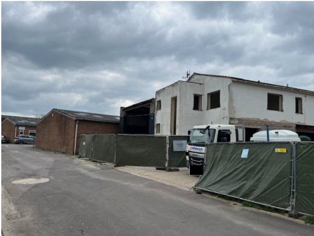
5. Side of Tesco site, opposite photograph. Photograph shows small business premises at the rear
